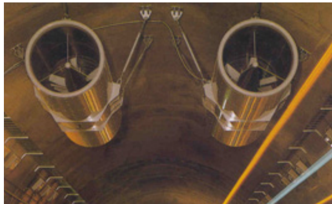
JET FAN Dia. 1,030~1,500 mm Power 30~55kW Outlet Speed 30m/s
