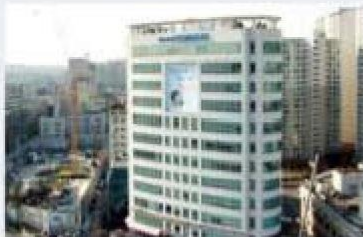
Main Business Center(13,500m 2 )
