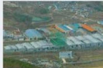
Cheong do factory(77,550m 2 )
