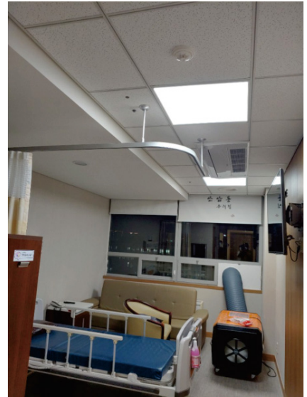
Installation completed in a hospital room (ARDC-1502)
