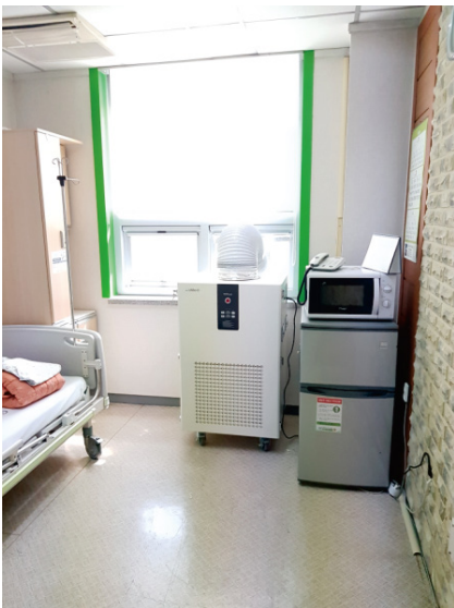
Installation completed in a hospital room (ARDC-1501)
